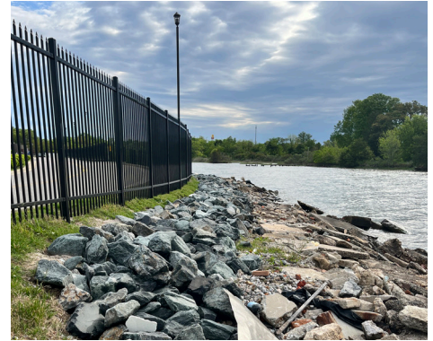
Hampton VAMC Perimeter Fence
